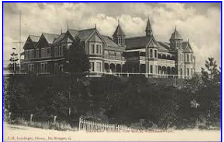
The building now showing the extensions added in 1897 (single story on the southern side), in 1899 (double story added on the south east side) and in 1901 (extra classrooms, laundry, pantry, storeroom, etc).
